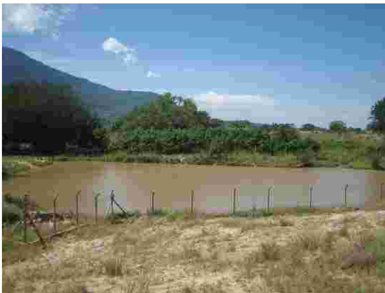
Figure 16: Water Valley Tank fenced with barbed wire to keep off livestock and children (Source: FAO/MAAIF, 2013 10 )
