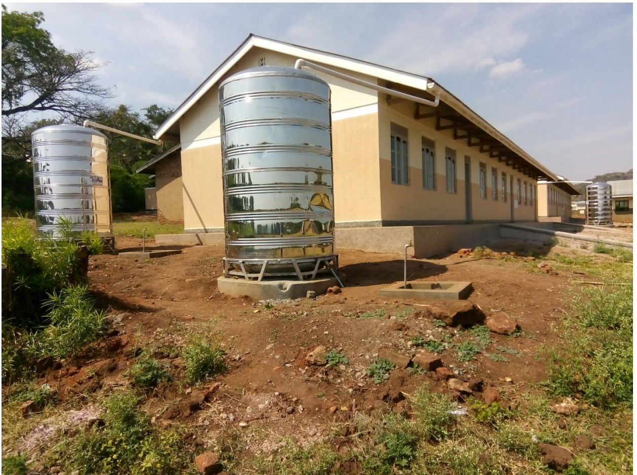
Classroom blocks built in one of the schools in a Refugee hosting communities with a fully fledged water harvesting system and latrine facilities.
